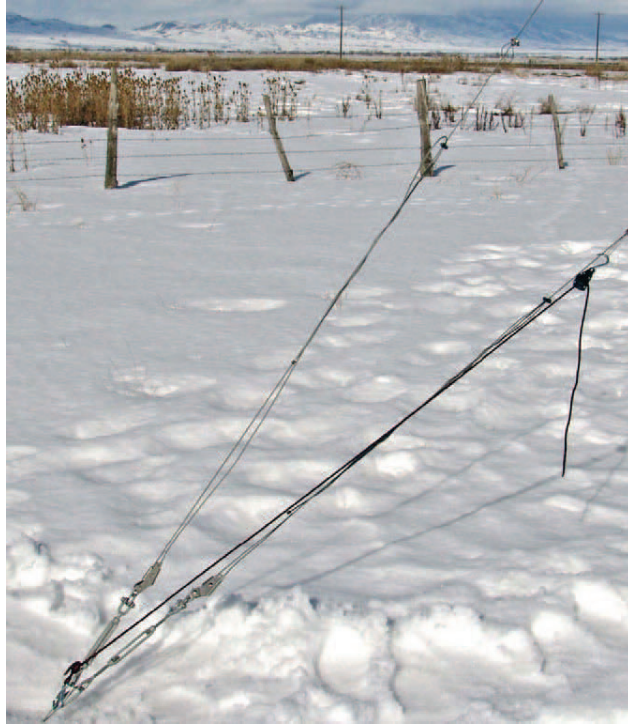
FIGURE 3-27. Rope ratchet assists assembly
