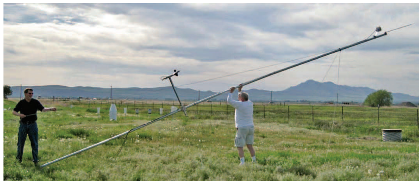
FIGURE 3-29. Raising the mast
