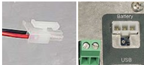
Figure 8-3. –ALK battery pack connection
