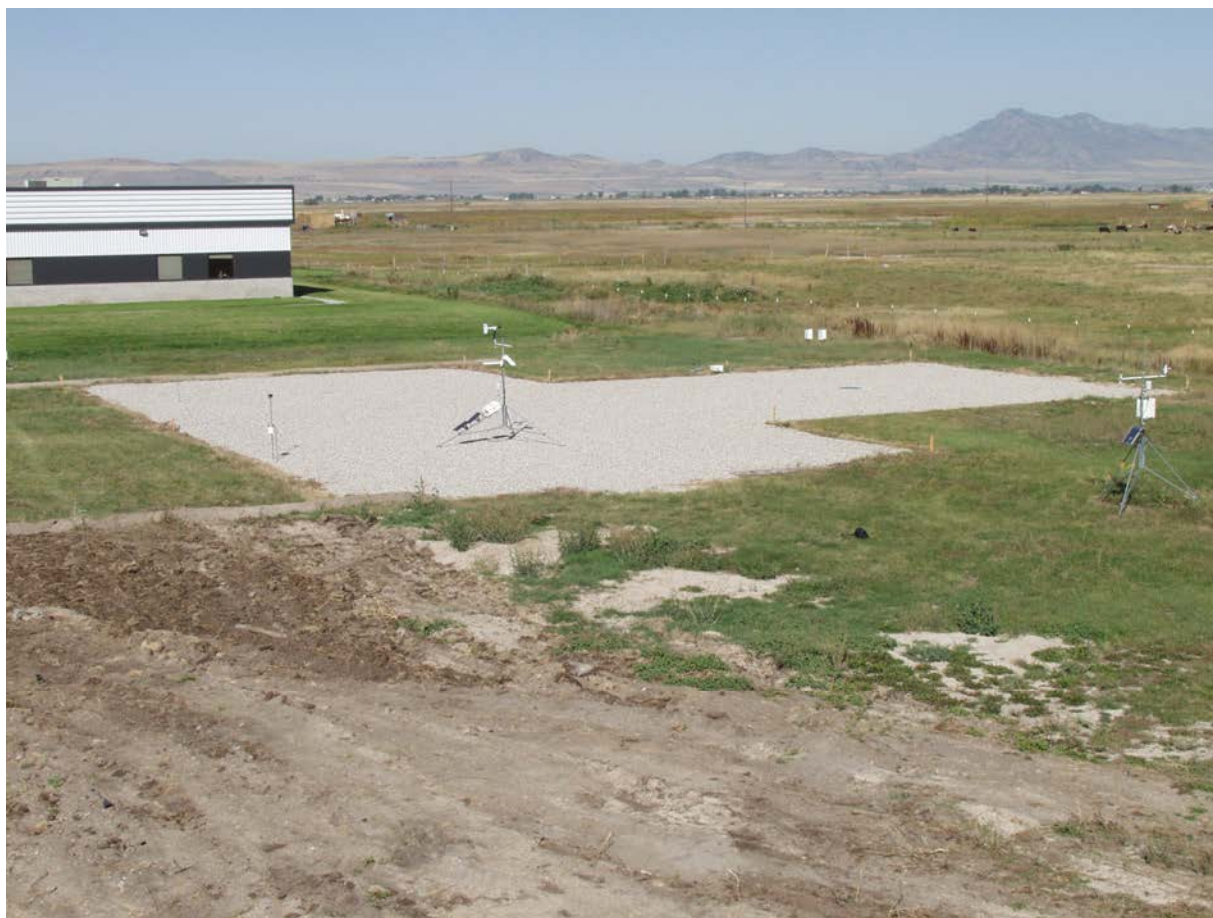
FIGURE 9. Campbell Scientific, Inc. electric field meter site correction facility
