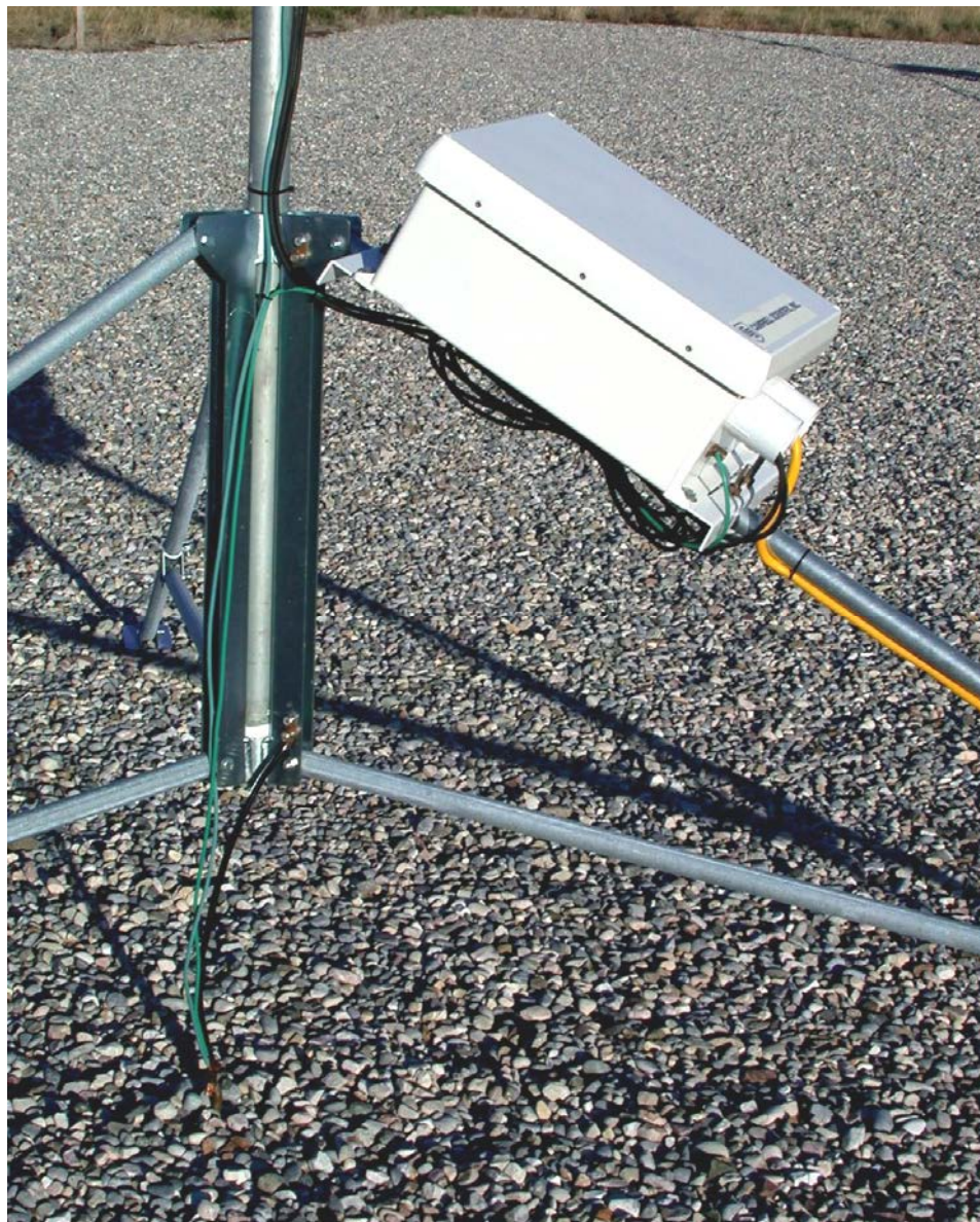
FIGURE H-4. Grounding the tripod and battery
