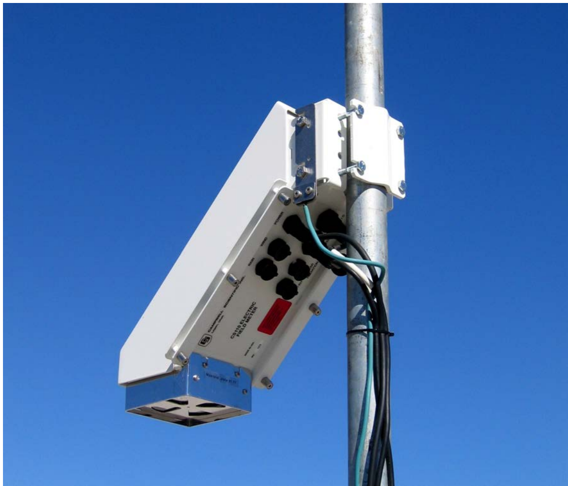
FIGURE H-3. Grounding the CS110 grounding strap
