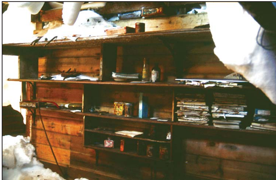
Snow and ice ingress represent serious threats to the structure and content of Mawson's Hut, as shown by this photo of icebound historic artifacts on Mawson's bookshelf.
