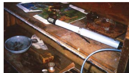
An HMP45C monitors internal RH and air temperature at Mawson's Hut.
