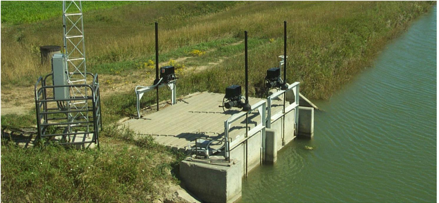
sensors, and gate actuators in combination with Campbell Scientific dataloggers (CR1000, CR850, and CR200X).
