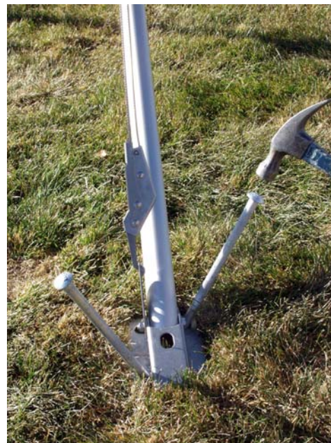
FIGURE 5-8. Staking the Tripod Feet
