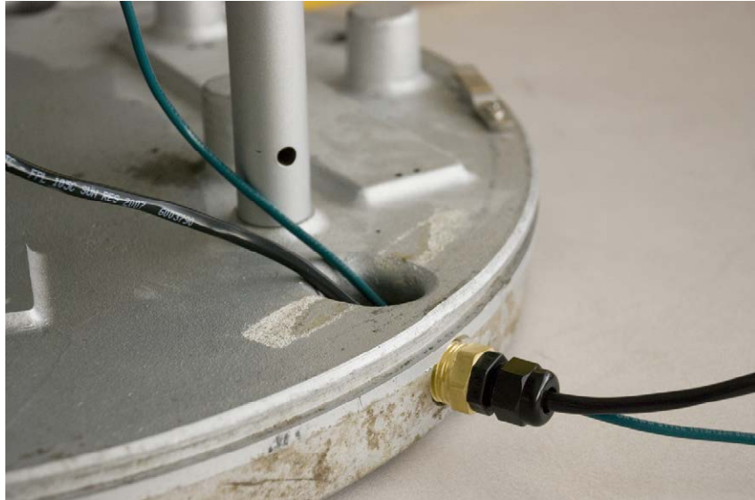
FIGURE 3.3-1. Solar panel cable and grounding wire routed through compression fitting of rain gauge base.
