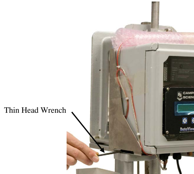
FIGURE 3.2-3. Tightening bolts to attach enclosure to the base.
