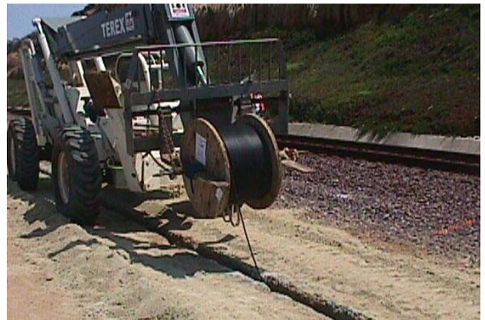
In Del Mar, California, a tractor-mounted trencher installed coaxial cable for monitoring slope stability using our TDR system.
