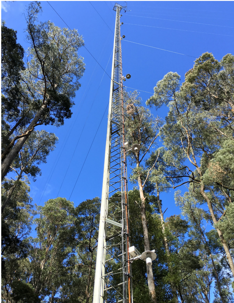
Looking up at the Warra Flux Tower. Several of the AP200 intakes can be seen. The CPEC200 is mounted at the top.
