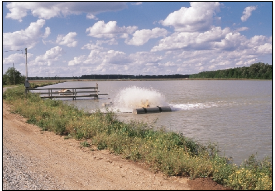
An automated aerator restores dissolved oxygen levels on one of many ponds at the Lee Catfish Farm in Mississippi. In addition to water conditions, current drawn by the aerator can also be monitored.
