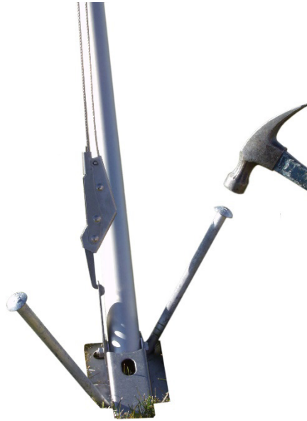
FIGURE 6-11. Staking the tripod feet
