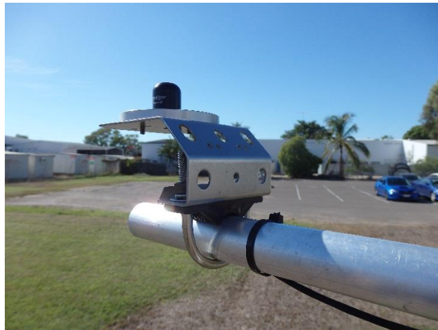
FIGURE 3-8. Installed SP-212 Pyranometer
