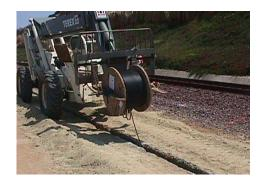
In Del Mar, California, a tractor-mounted trencher installed coaxial cable for monitoring slope stability using our TDR system.
