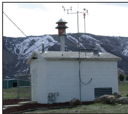
A system monitors water and meteorological parameters at a pump control site for the Mantua, UT, water system
