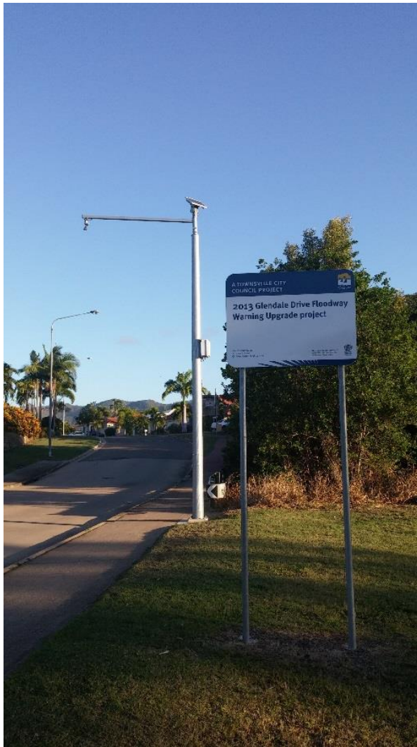
Figure 6: Radar Roadway Flood Monitoring System installed at the Glendale Drive floodway in Townsville.
