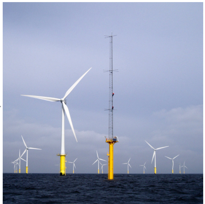
A Campbell Scientific datalogging system monitors this offshore wind farm located between Rhyl and Prestatyn in North Wales at about 7 to 8 km out to sea.
