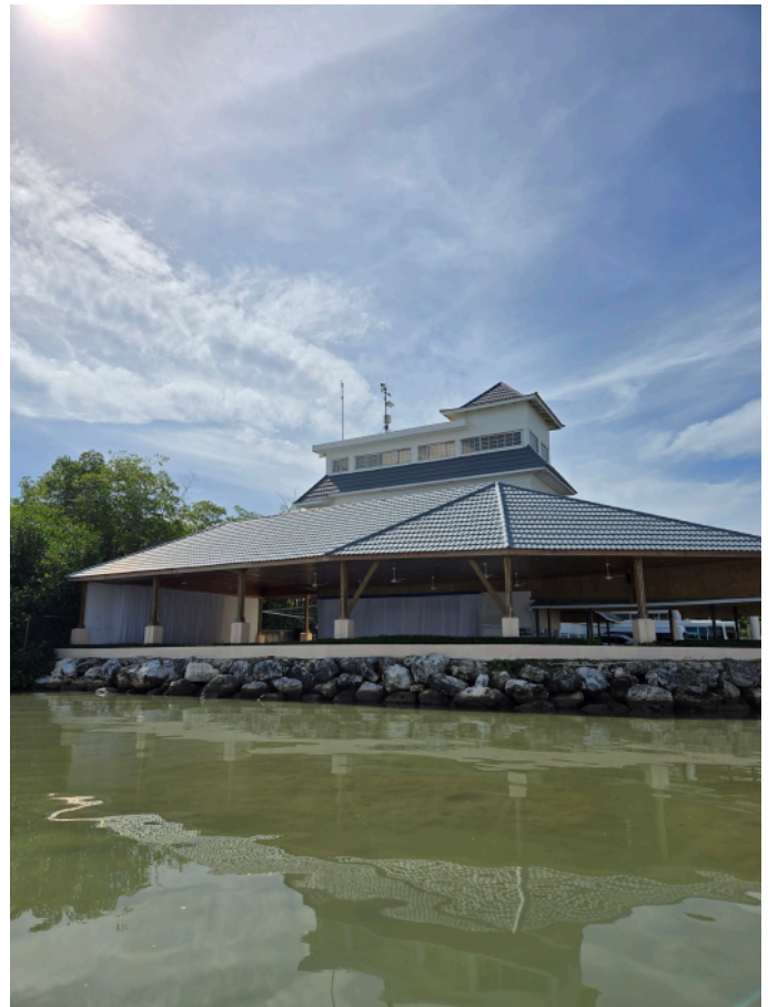
The automated weather station bolted to the roof of the Glistening Waters Hotel
