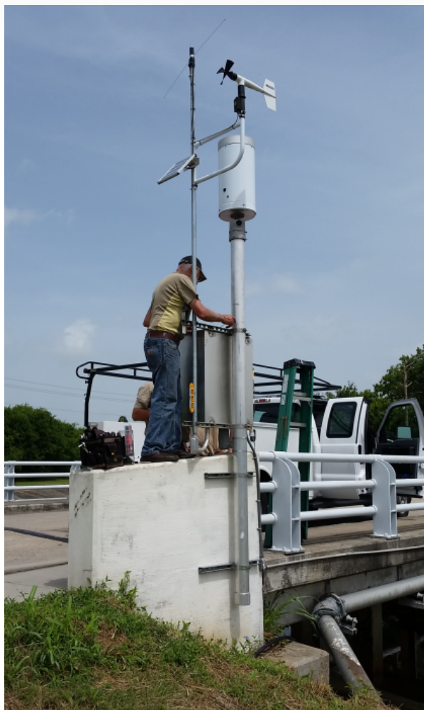
Installing Campbell system for HCFCF
