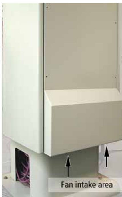
Fig. 27: Fans inlet. Remove snow, sedimentation,...
