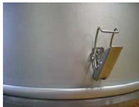
FIGURE 6—6. Gauge cover. Close-up of clamp
