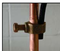
Figure 19: The #4 cable connected to the ground rod.
