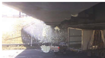
Virginia Avenue bridge impact event
