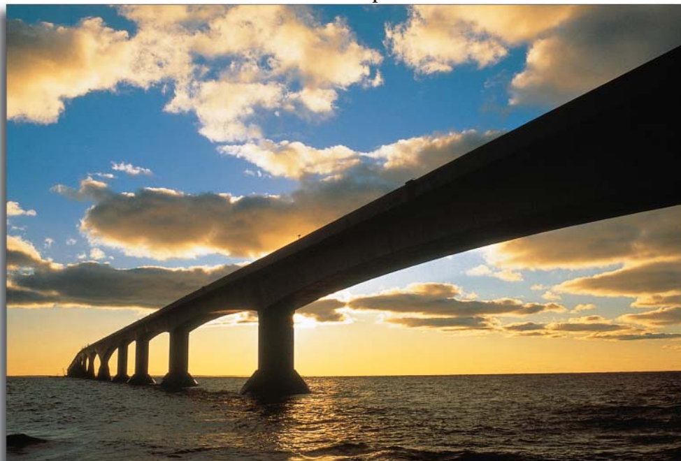
Campbell Scientific data acquisition systems make reliable structural measurements, even in harsh, remote environments. The 13 km Confederation Bridge that connects Prince Edward Island with mainland Canada was instrumented to document strain during ice impacts and to observe weather.
