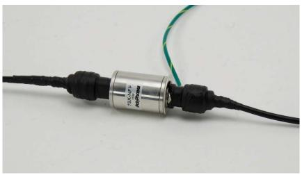
7. Wrap both connections a second time, contiguous with the surge protector, from end to end. Extend the ground wire from the wrapping parallel to an antenna cable.
