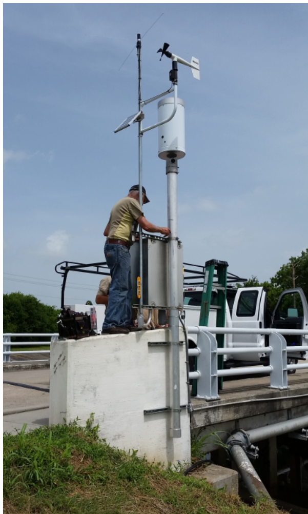
Installing Campbell system for HCFCD
