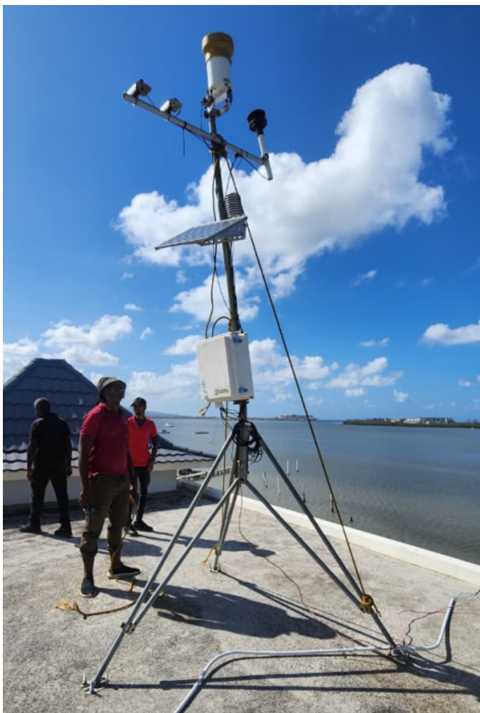
The automated weather station bolted to the roof of the Glistening Waters Hotel
