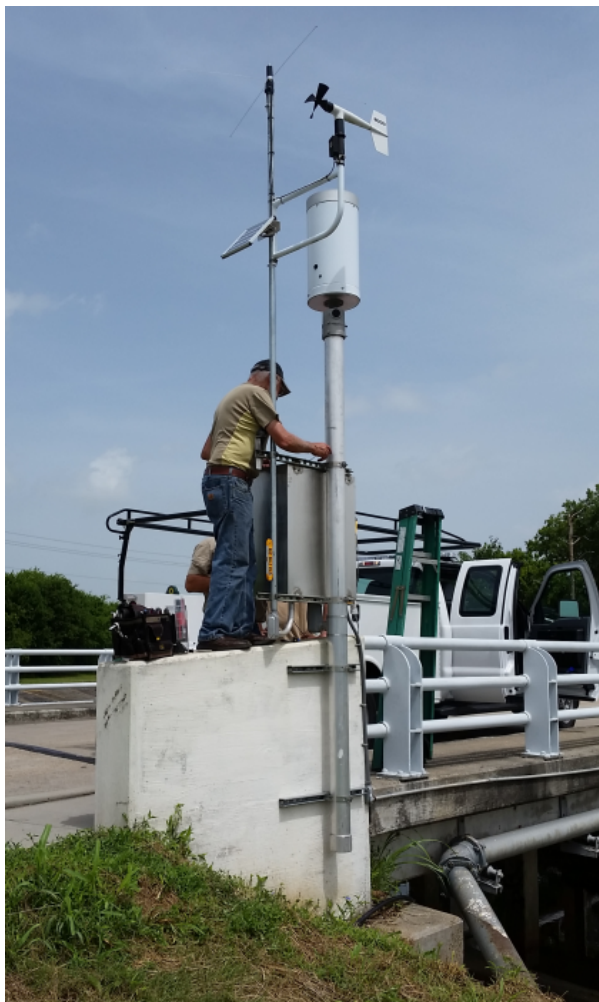
Installing Campbell system for HCFCD
