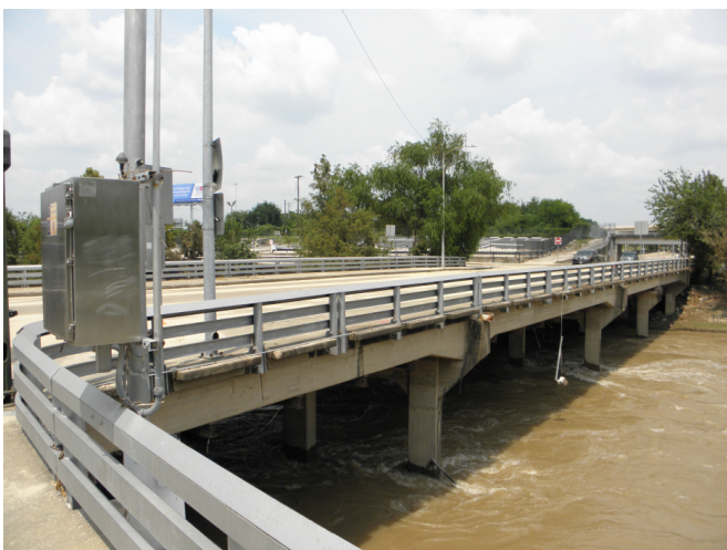
High water from Hurricane Harvey
