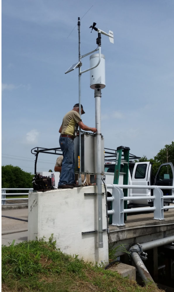
Installing Campbell system for HCFCD
