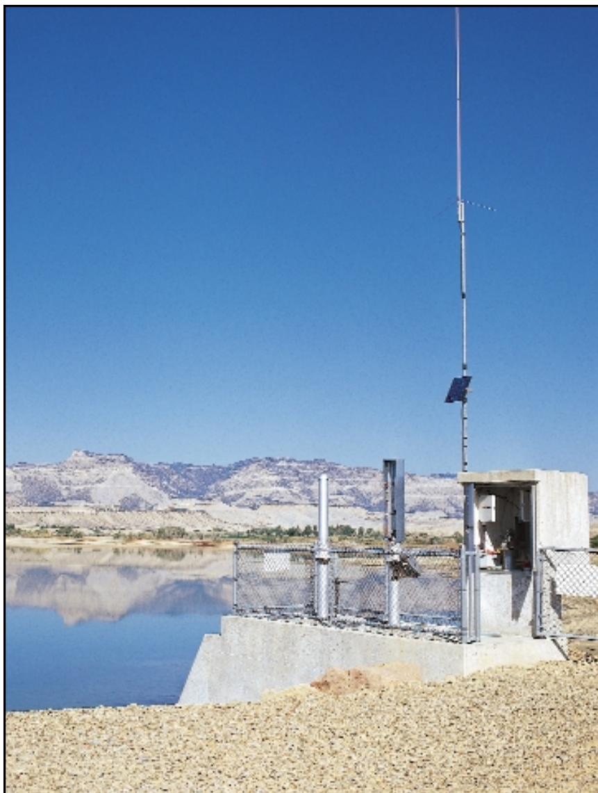
A CR10 accessed by RF telemetry at North Huntington Reservoir allows the district manager to control the headgate from Castle Dale, 13 miles away.
