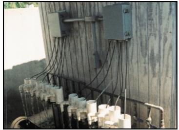
Rather than deal with the added expense of extra cable lengths for 12 individual dissolved oxygen probes, Stolt Sea Farm devised a system in which water continuously flows from the tanks through PVC pipe to sensors at the monitoring station.
