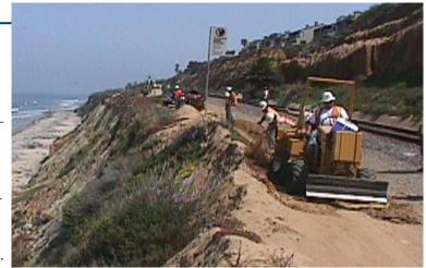
data indicated a deformed or broken cable, an alert signal consisting of 5 Vdc was applied to a wire monitored by the CR23X Micrologger<sup>®</sup> at the central control and monitoring unit. There, an automated telephone dialer notified railway personnel of possible bluff movement. Personnel could then contact the system by telephone and determine the location of the cable deformation so that a safety inspection of the bluff and track could be made.
