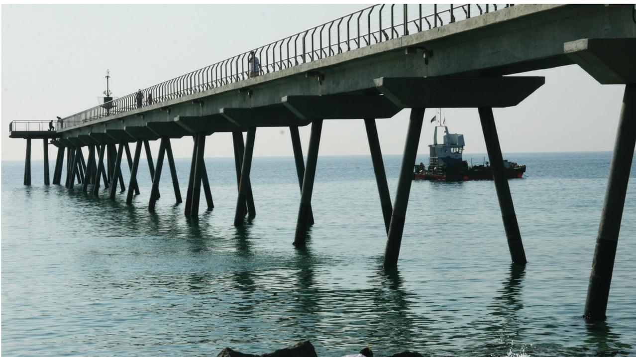
The pier is 6m above the water and extends 250m into the sea. The water below the monitoring station is around 12m deep.
