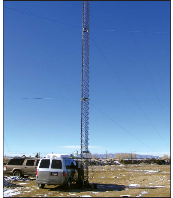
An 82-meter (270 ft) IsoTruss tower fitted with one CR1000, two LLAC4s and nine wind speed sensors profiles wind at the mouth of Spanish Fork Canyon, Utah.
