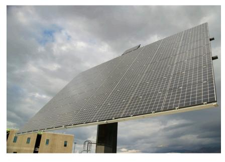
a stationary station with a reference solar panel, and then instrumented that reference station and the tracking solar array with temperature sensors, pyranometers, and power-output sensors. We will be able to measure the output of a panel on the tracker tower
