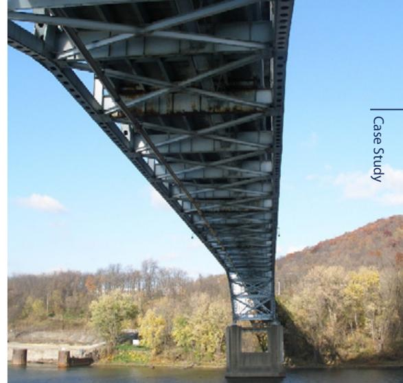
for about three months. During the monitoring period, the CR9000X was triggered to record high-speed, time-history data when high-stress events were detected. In this way, data records were obtained for crossings of the heaviest vehicles.
