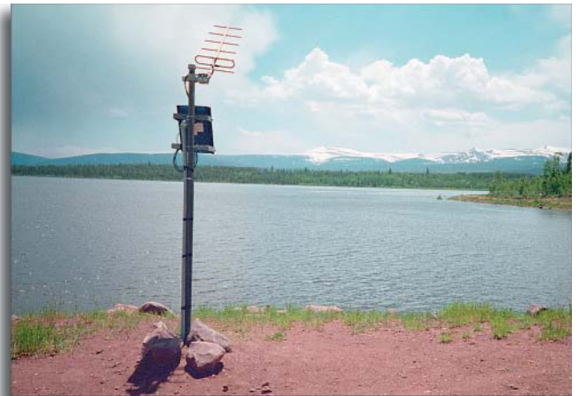
Monitoring systems at the Long Park Dam (Daggett Co., Utah) helped identify and prevent an imminent dam failure.
