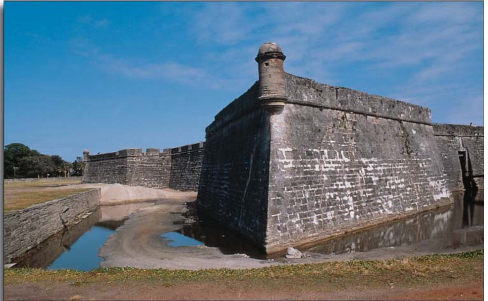
Cracks in the walls of Castillo de San Marcos, Florida were instrumented to determine their genesis and the best course for corrective action.
