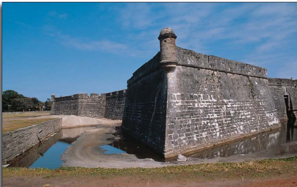
A preservation project at Castillo de San Marcos, St. Augustine, FL involves monitoring cracks in three dimensions, the tilt of the large segments between the major cracks, change of soil moisture within the bastion, and weather conditions at the site.
