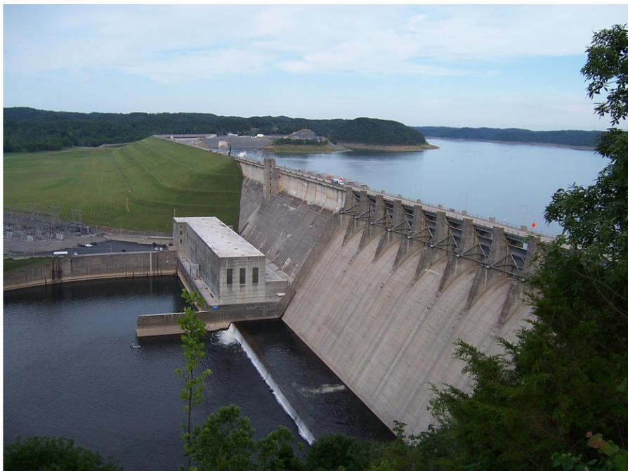
The Wolf Creek Dam near Jamestown, Kentucky, was constructed partially as a regular concrete hydroelectric dam, but mostly as an earth-fill embankment structure. Finished in 1950, within 20 years it developed serious reservoir seepage problems. Several repair projects had a degree of success at stemming the flow, but in recent years managers decided that resurging seepage at the dam constituted an emergency situation.
