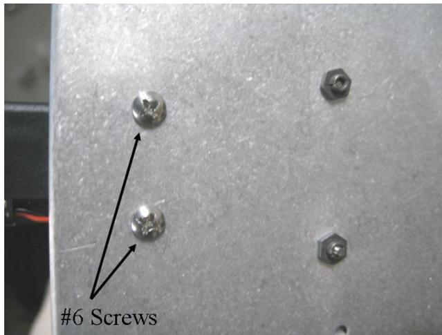
FIGURE J-8. Self-tapping screws attaching pump to metal box
