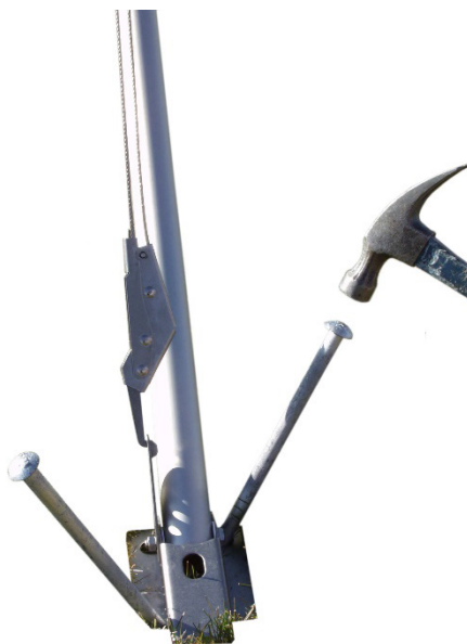
FIGURE 6-11. Staking the tripod feet
