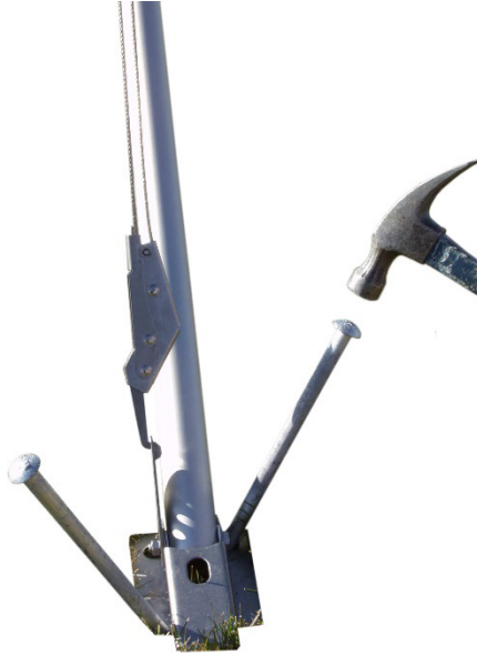
FIGURE 6-10. Staking the tripod feet
