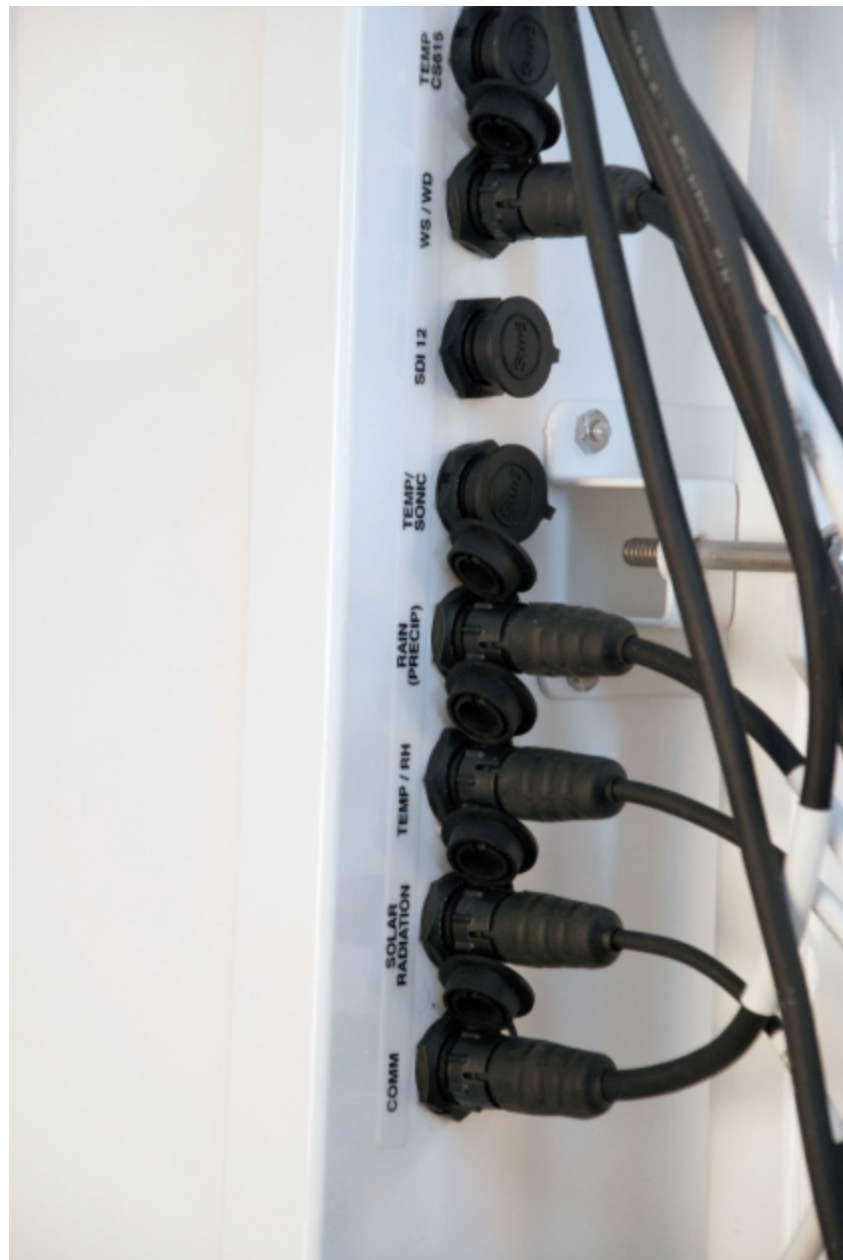
FIGURE 6-21. Connecting sensor cabling to enclosure
