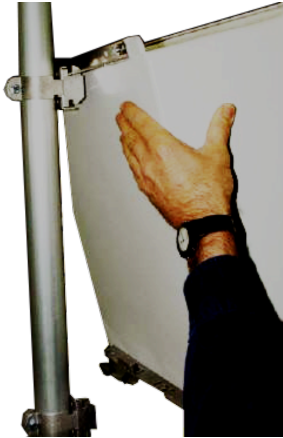
FIGURE C-6. Top clamp hook side up
