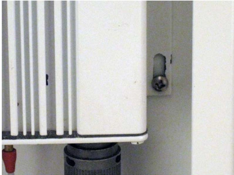
*Figure 2. Proper mounting position of the electronics box.*
