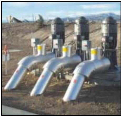
The operation of irrigation pumps is controlled by a datalogger digital I/O ports while flags trigger alarm call-outs to cellphones. Water Reuse Facility, Silver Springs, NV, USA
