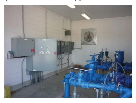
pumps and valves, with each town controlling the valves to allow or disallow the water flowing to the other.
