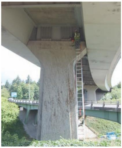
Kamal's Bridge in Tualatin is a steel box-girder bridge with four spans crossing Interstate 5. ODOT sought to improve the monitoring of the bridge's structural re-
