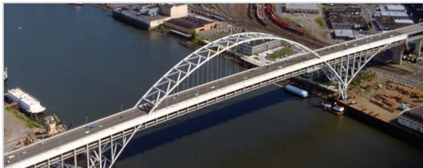
EMS designed and installed a monitoring system of eight CR800 dataloggers and a variety of sensors (including 64 sensors measuring strain and surface temperature) along the tie girders on both sides of the bridge. This system monitors the stress cycles in the tie girders due to thermal loading.
