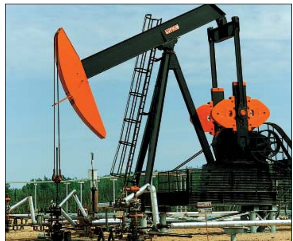
Wide operating temperature ranges, solar-, AC- or battery-powered operation, wireless communications, and reliable performance make our systems ideal for unattended monitoring.
