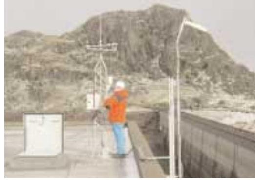
The Campbell AWS on the Stwlan dam in Wales
