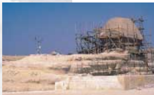
Weather measurements on the Sphinx provide input for its preservation.
