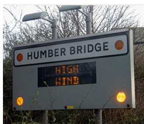
Wind warning systems can be directly controlled by a weather station
